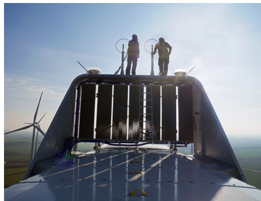
View from the nacelle of the Kraasa VII turbine
